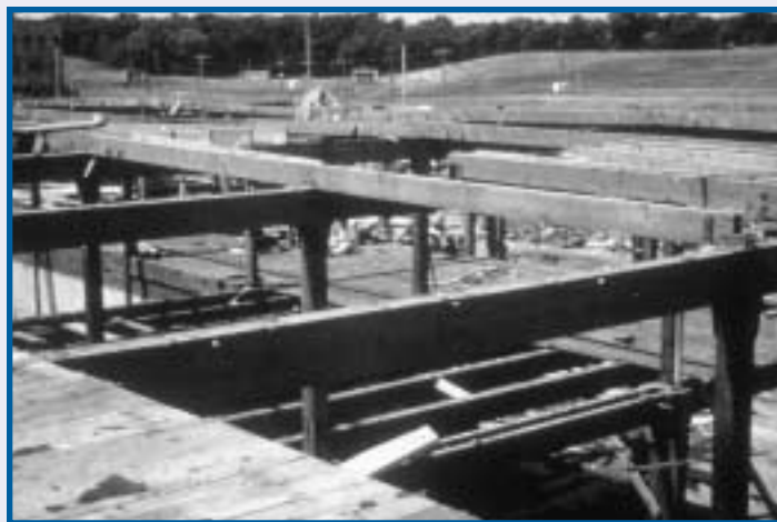
Deconstruction at the Twin Cities Arsenal, St. Paul, Minnesota.
