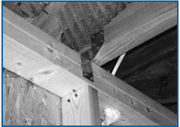
Residential wall-to-roof connector to resist uplift forces from high winds.
