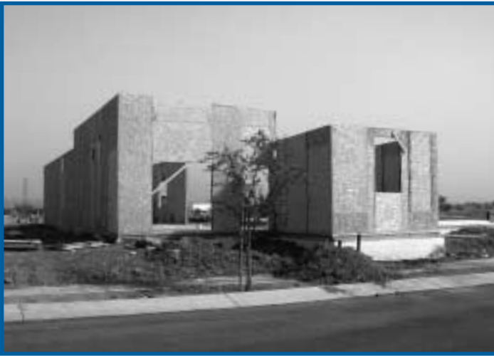
Structural insulated wall panels are an example of the innovative systems that were demonstrated at the Hands-On BUILDER workshop in Tucson, Arizona.
